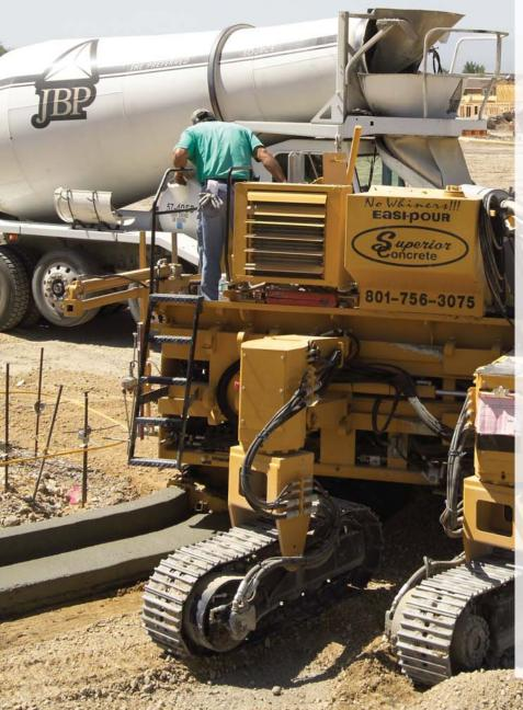
Slipform paver offers turning radius of less than 2 ft for increased worksite versatility and efficiency.
