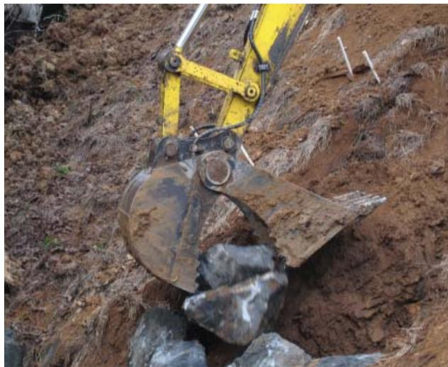
restore stream habitats. He uses a unique Kobelco 200 excavator with an extendable dipper stick to rebuild washed out road banks and stream habitats. The extendable dipper stick allows him to do more work
